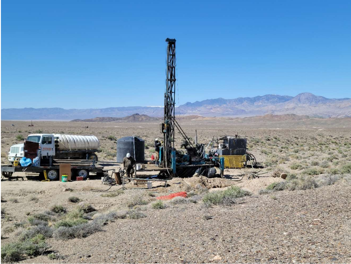
Figure 10-2: Phase VI Drilling: LF-70 Rig on CVZ-74
